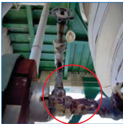
Corrosion under insulation
